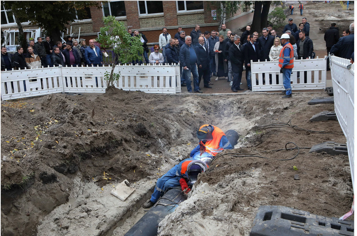
Kyivteploenerho workers replace the pipes of the capital's heat network that were damaged by Russian missile strikes in Kyiv, Ukraine, on Sept. 20. Tarasov Volodymyr—Ukrinform/ABACA/Reuters
